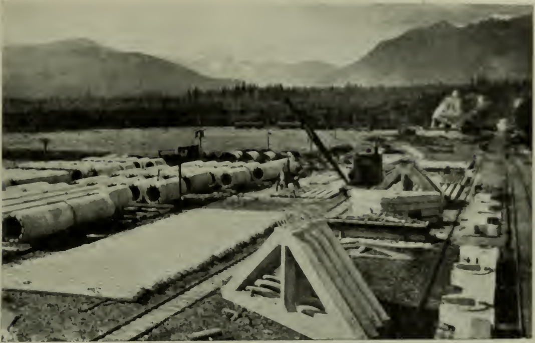
VIEW OF STORAGE YARD FOR PRE-CAST UNITS.
